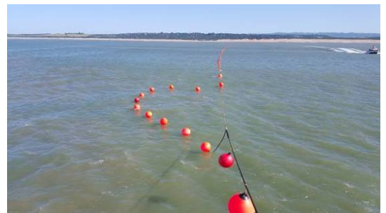
Plate 7 Bringing the cable to shore from the cable laying vessel. The cable is buoyed off and pulled to shore with smaller vessels
