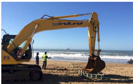
Plate 8 Landing of the cable on shore. Similar works will be undertaken for the landing of the 2AFRICA/GERA (East) Cable System in Port Elizabeth.
