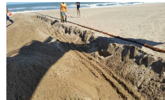
Plate 8 Landing of the cable on shore. Similar works will be undertaken for the landing of the 2AFRICA/GERA (East) Cable System in Port Elizabeth.
